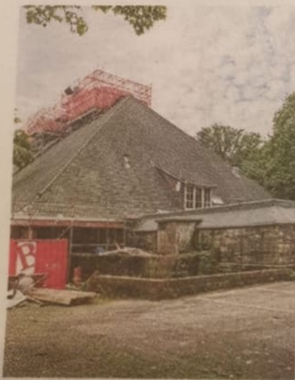
De bunker in de steigers.
